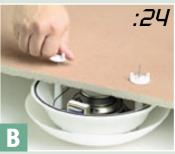
Wide-based wing nuts secure the speaker assembly to the ceiling tile.
