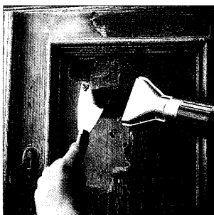
z.B. Removing paint and lacquer
